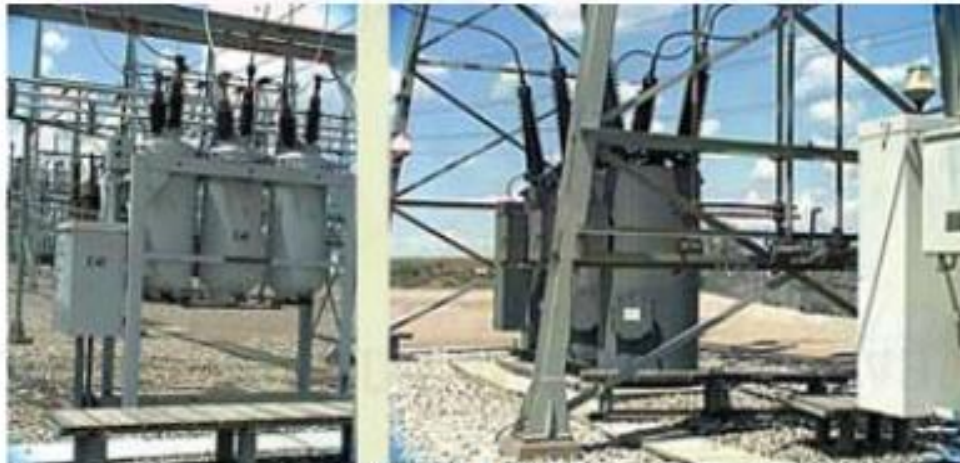
Oil Circuit Breakers
